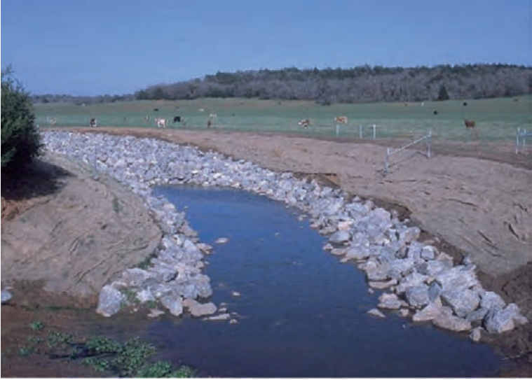
Plate 44 Grade stabilization structures are established along drainageways to prevent gully erosion (Courtesy USDA-NRCS)
