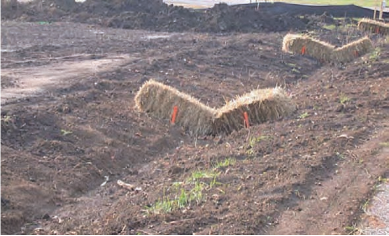
Plate 48 Straw bales are used to stabilize waterways (Courtesy Ryan Bartels)
